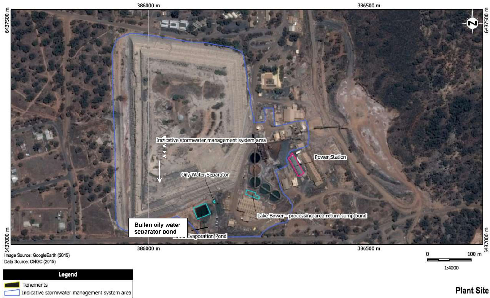
Figure 2 Emission points and containment infrastructure defined in Tables 1.3.1 and 2.2.1
