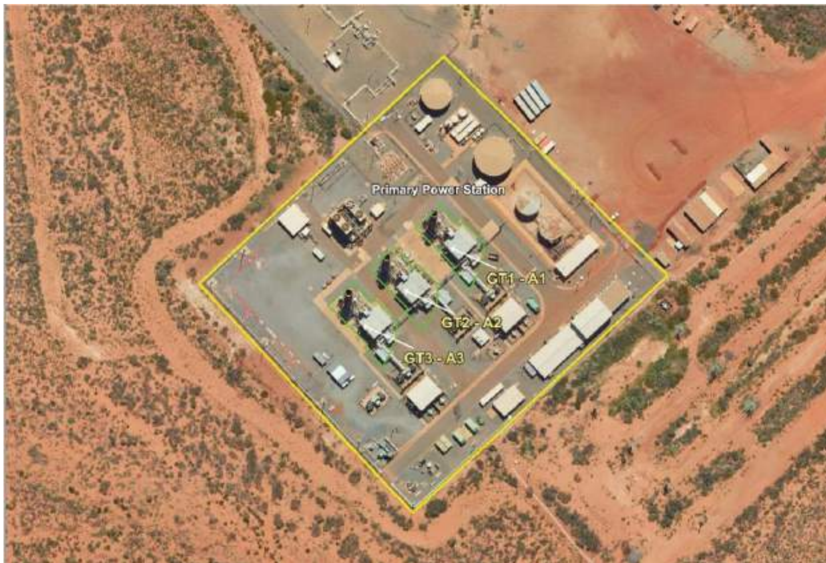
Figure 11: Primary Power Station Air Emission Points A1 – A15. Air Monitoring Points A1 – A3
