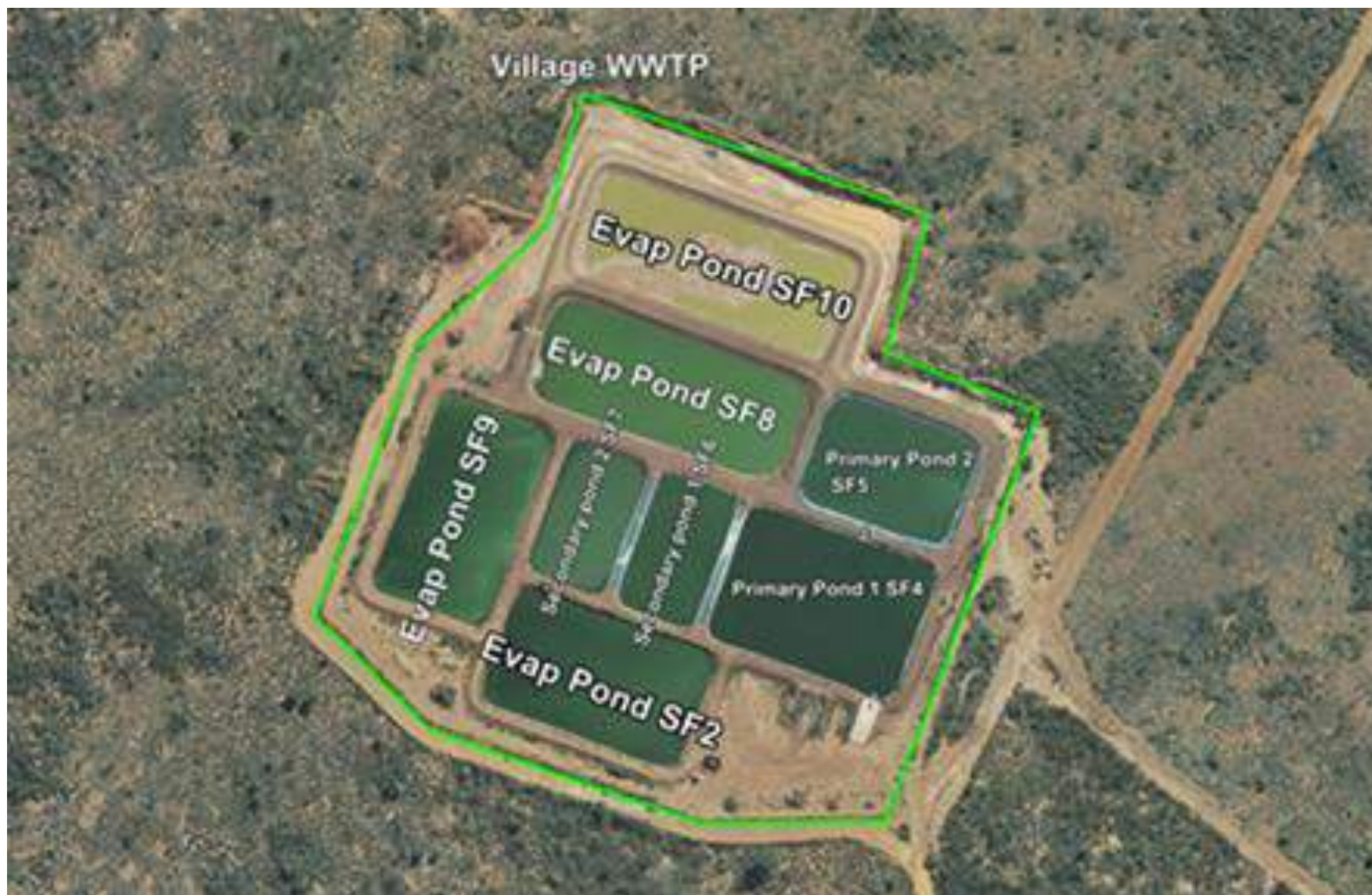
Figure 8:Village WWTP Primary, Secondary and Evaporation Ponds (zoomed extent)
