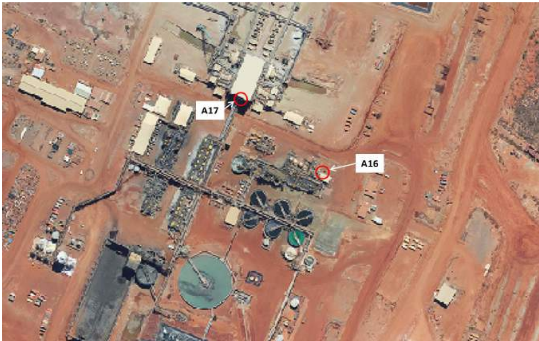
Figure 12: Carbon Regeneration and Gold Room Air Emission Points A16 and A17.
