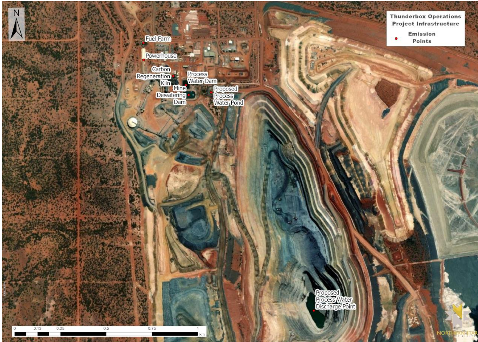
Figure 2 Process Water Pond emergency discharge point (Thunderbox Pit)
