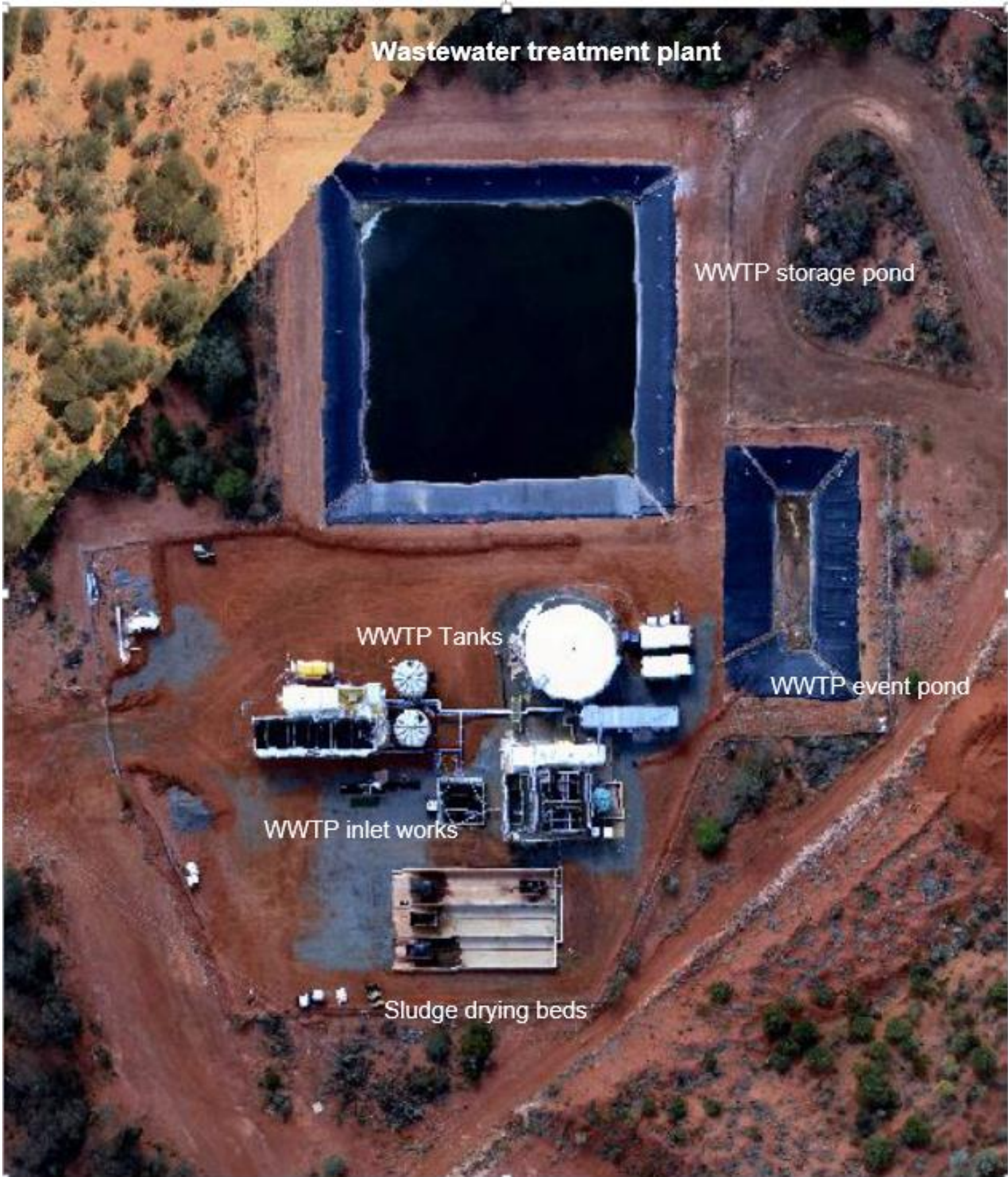
Figure 4: Wastewater treatment plant infrastructure
