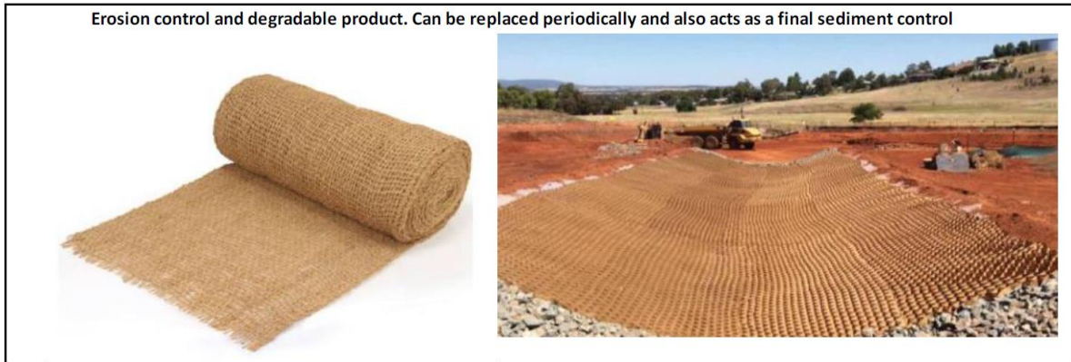
Figure 4: Geofabric installation details
