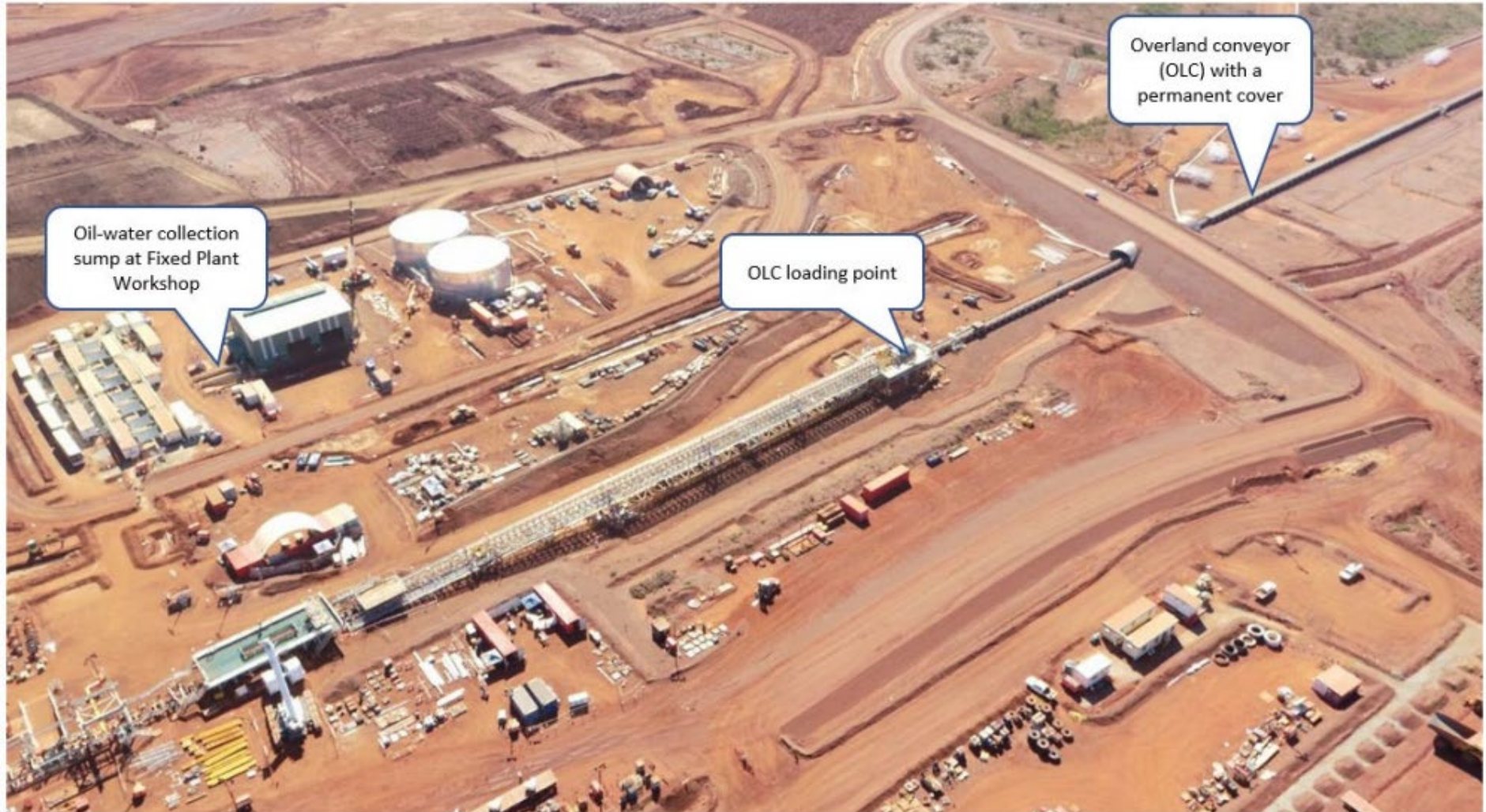
Figure 13: WTS S2 Conveyor
