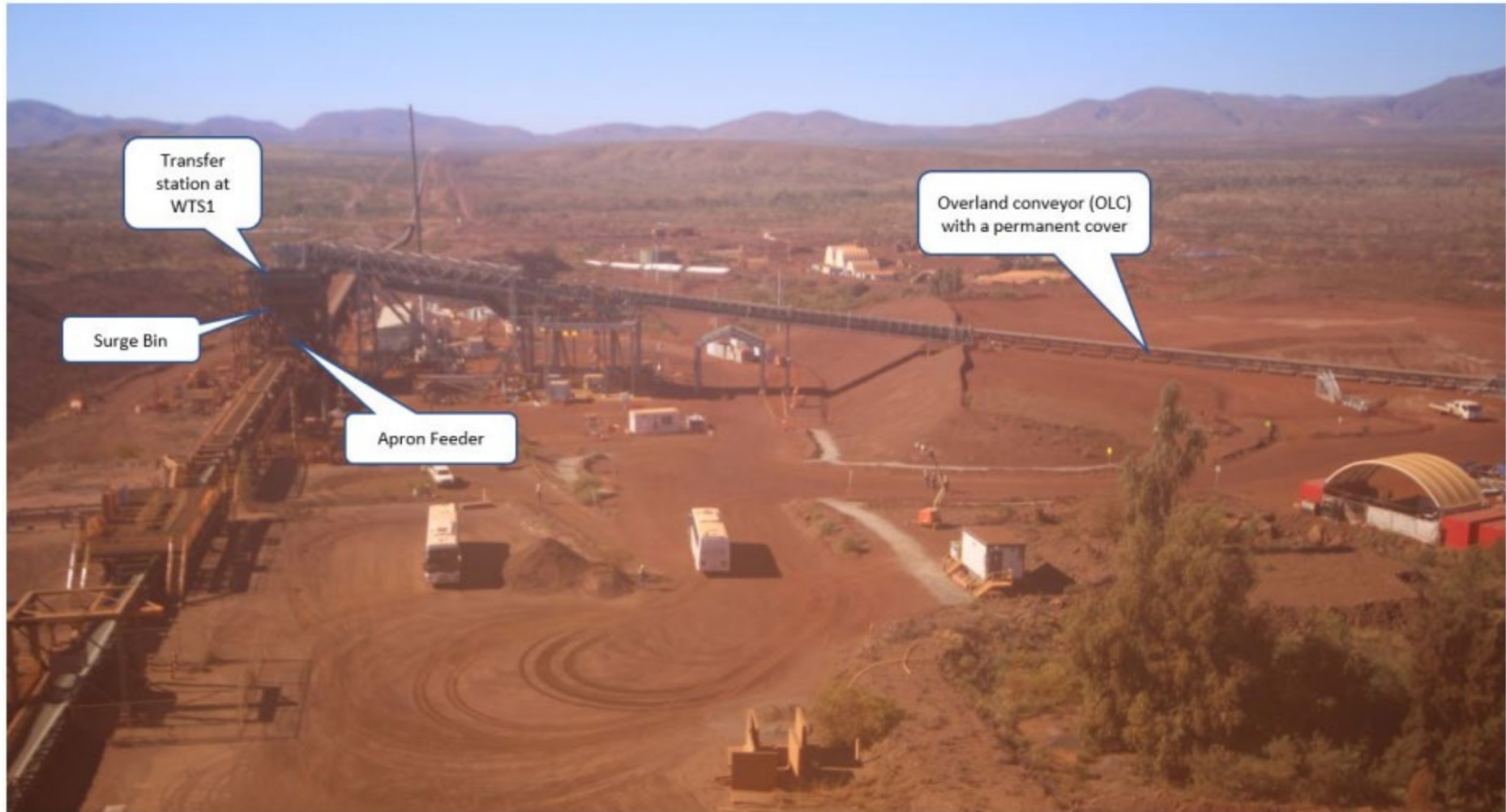
Figure 14: Processing Facility – WTS S1 end
