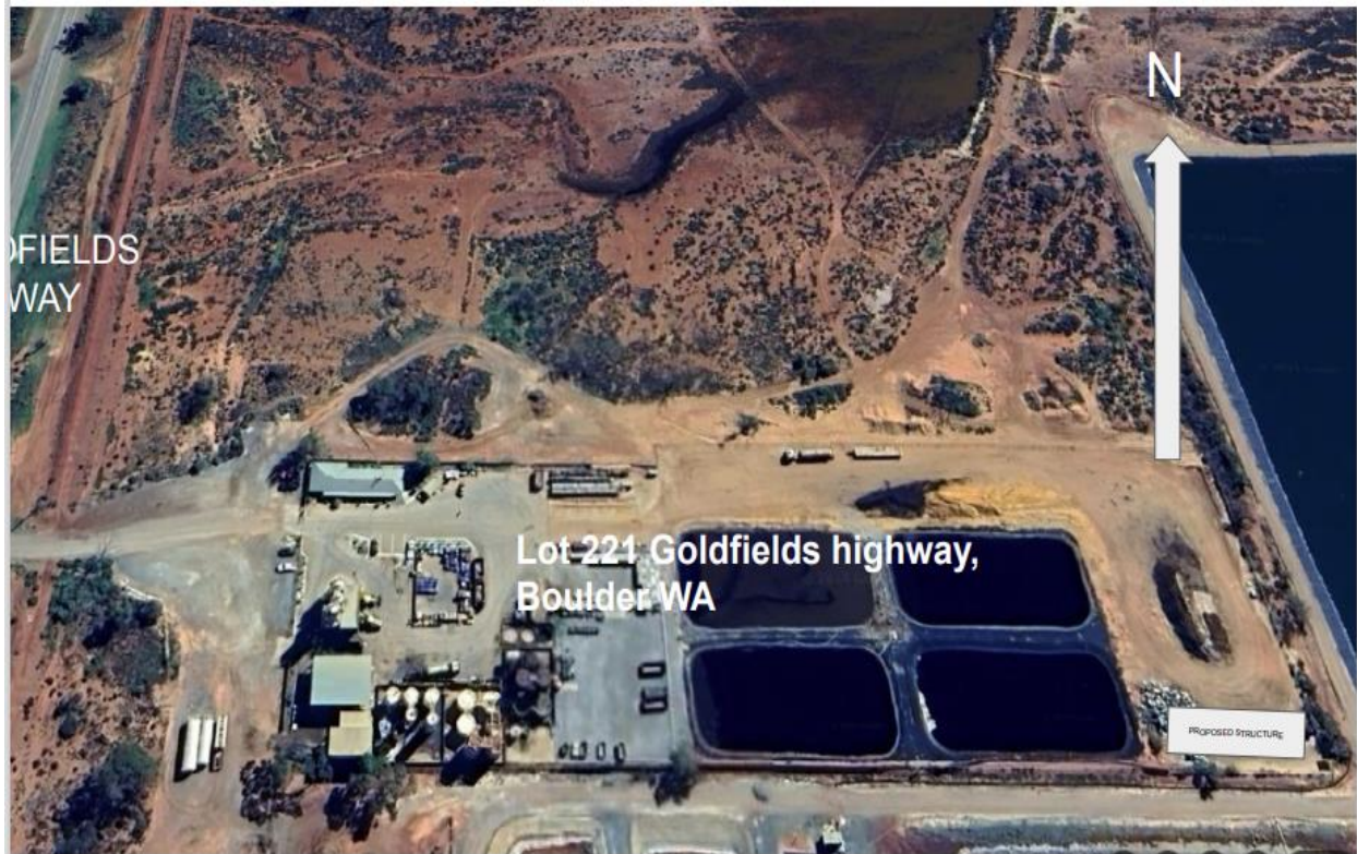
Figure 5: Location of the concrete hardstand transfer pad as outlined in white
