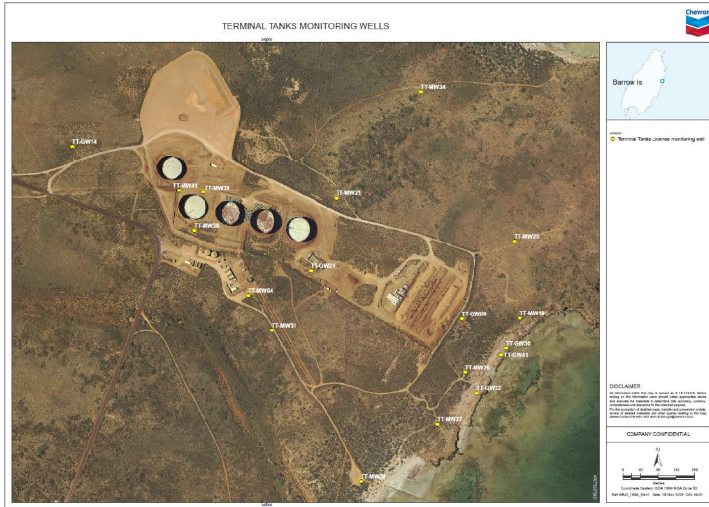
Figure 6: Terminal Tanks, Terminal Tank Stormwater Receiver monitoring well locations
