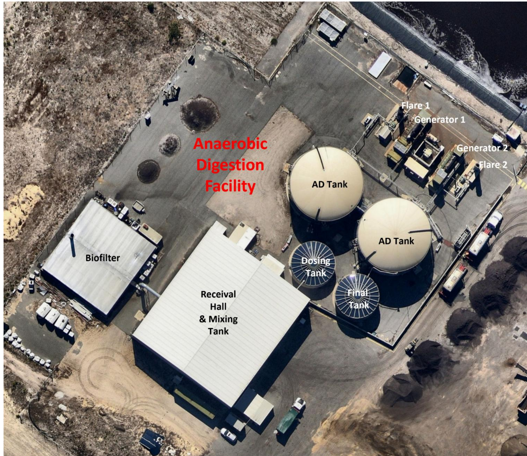
Figure 3: Anaerobic Digestion Facility
