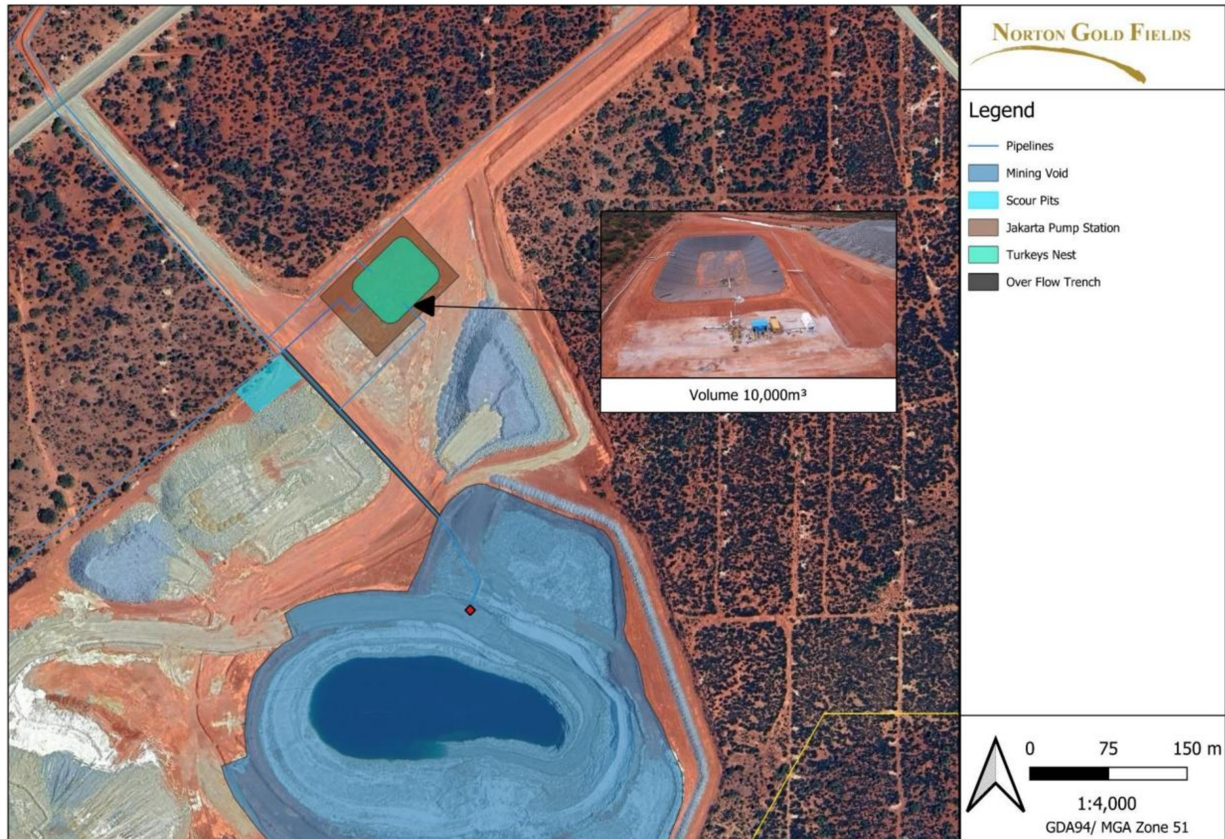
Figure 4: Jakarta turkey's nest/pump station
