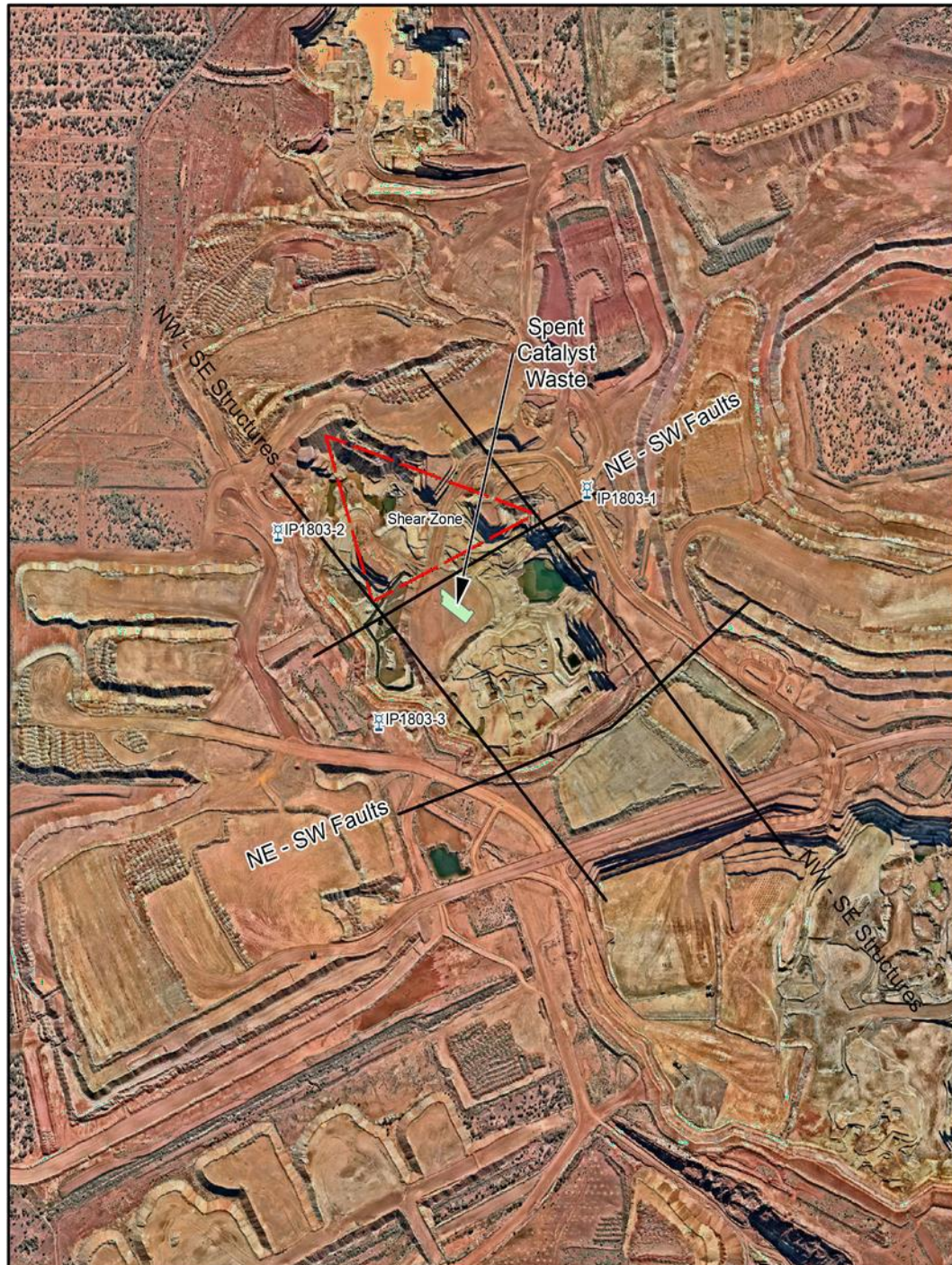
Figure 22: Disposal of spent vanadium catalyst
