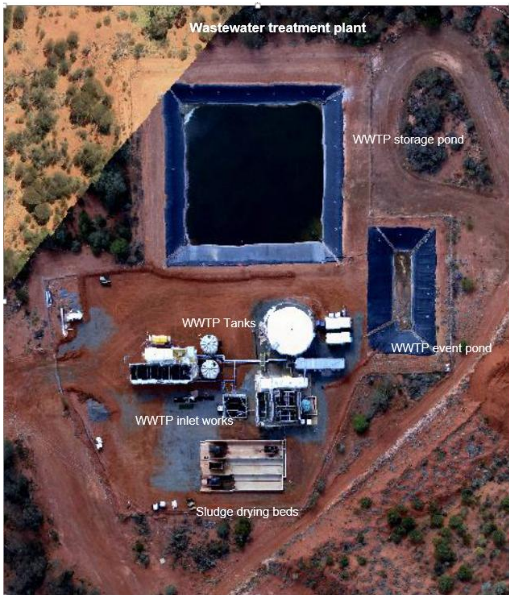
Figure 4: Wastewater treatment plant infrastructure
