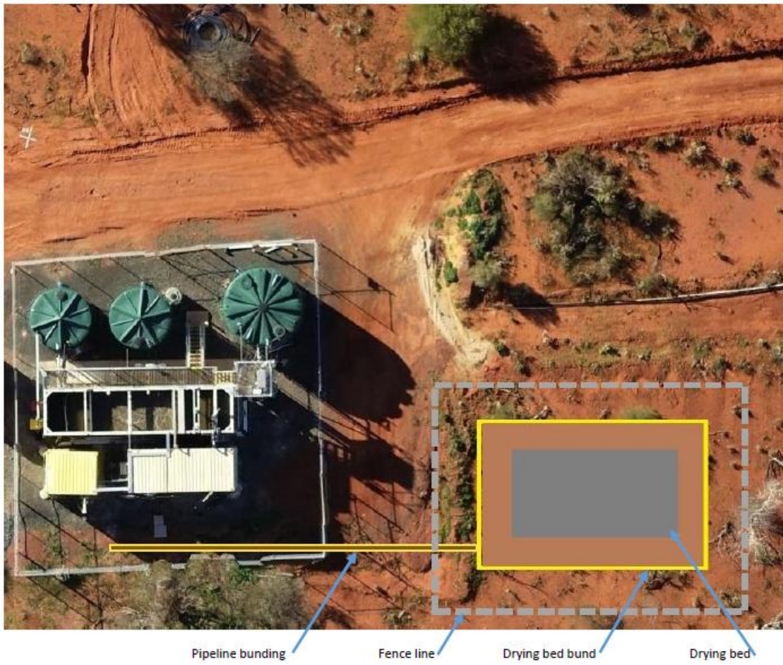
Figure 10: Sludge drying bed location.
